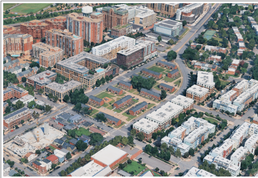
Figure 1. Samuel Madden Homes Redevelopment Site
